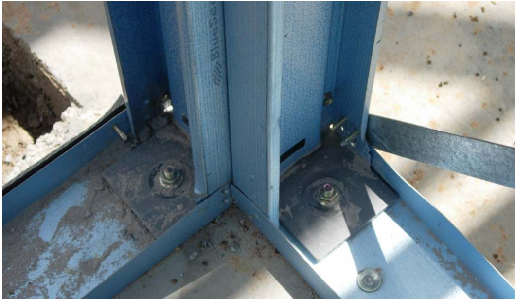
Figure 6: Well detailed bottom plate anchorage showing heavy washers located as close as possible to the end studs.
