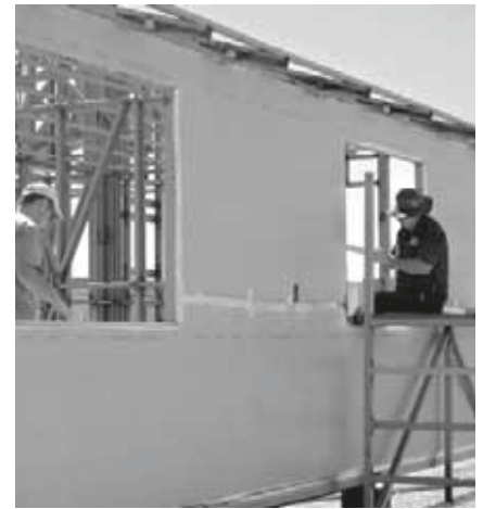
Air-Cell Permishield used as building wrap.
