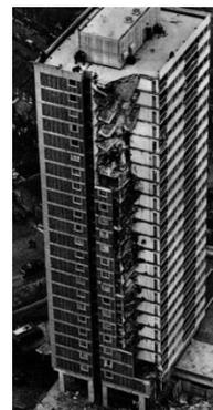
**Figure 1 Ronan Pt failure due to gas explosion**
