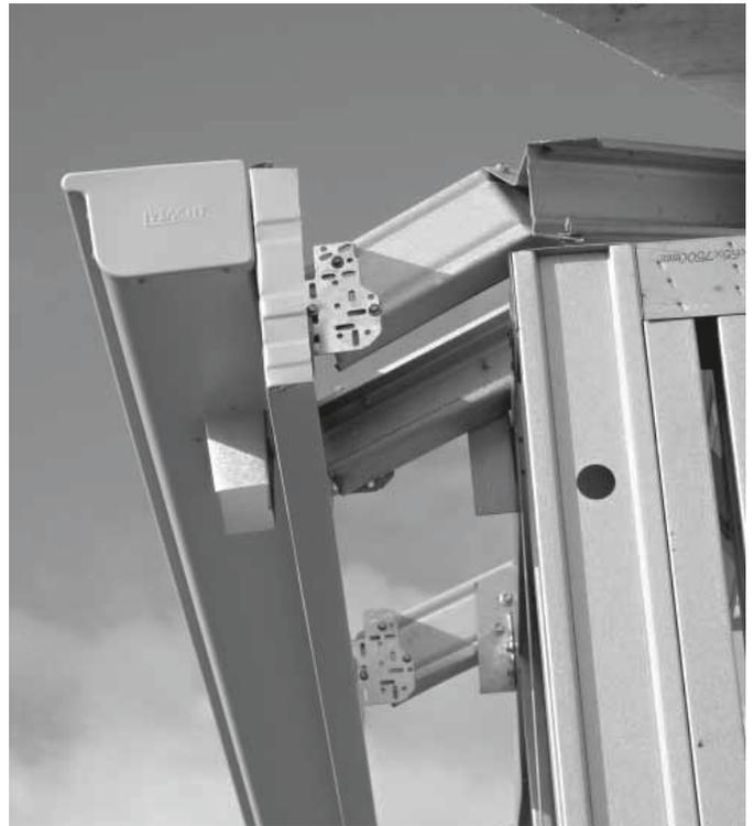
provide protection without the need for grommets. Manufacturers usually provide multiple holes in studs and plates to make wiring and plumbing easier for contractors.
