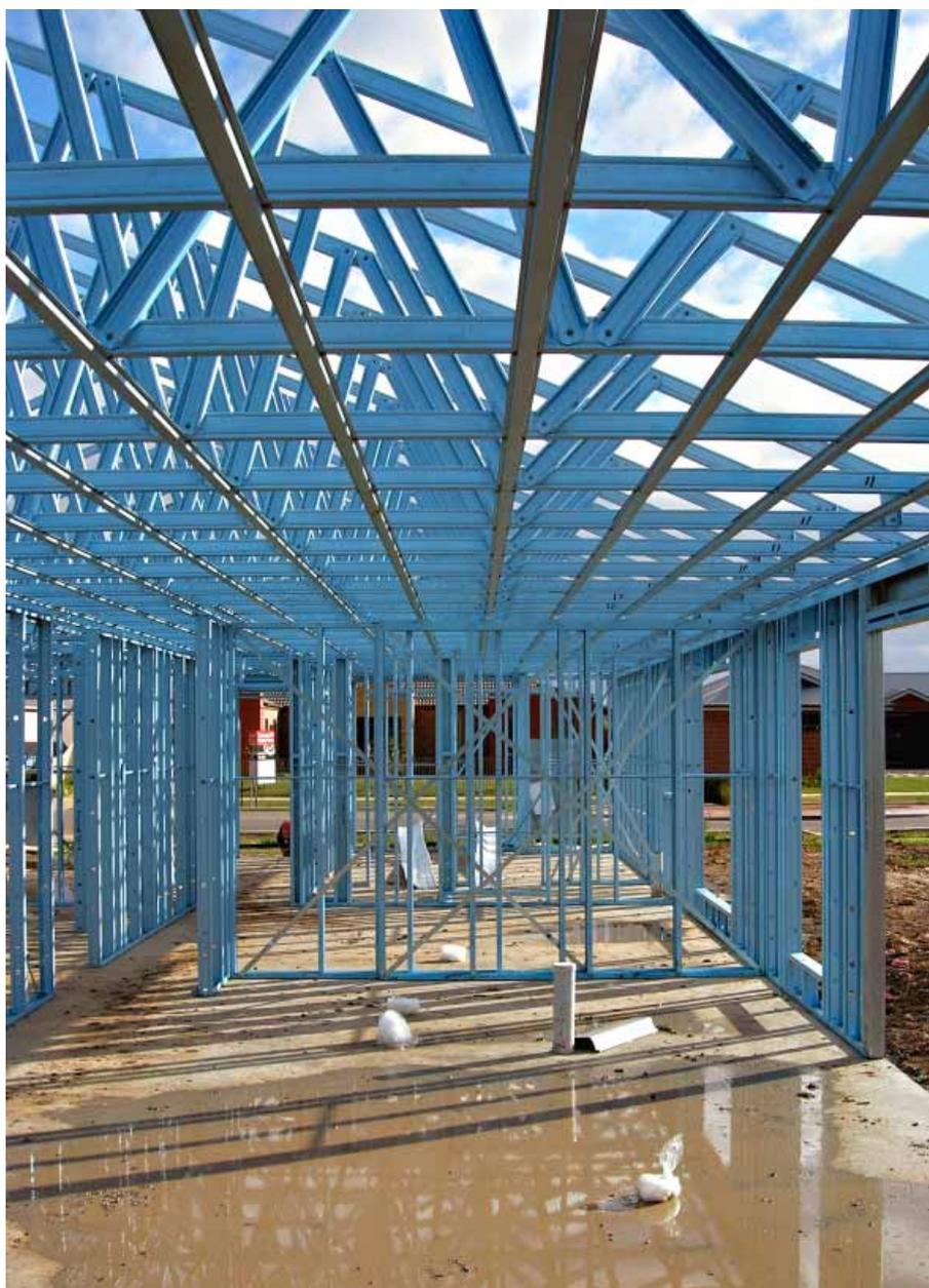
Your steel frame is now structurally complete and ready to support the roofing, cladding, lining, fit out components and services that will turn it into a dwelling. All of these items have particular fixing requirements to ensure a sound, serviceable and aesthetically pleasing finish. If you have built the structure carefully and accurately, you can expect few problems in the finishing stages.
